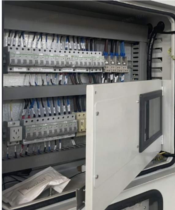
Figure 6- 2 Installation of BMS Display and Control
